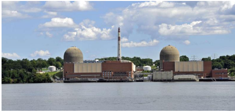
Figure 1. The Indian Point Generating Station in Buchanan, NY
